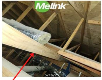
Return duct for this RTU was incomplete. The diffuser was not installed.
